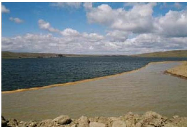
Figur 9.8 Siltgardin (Geomembran, 2006)
